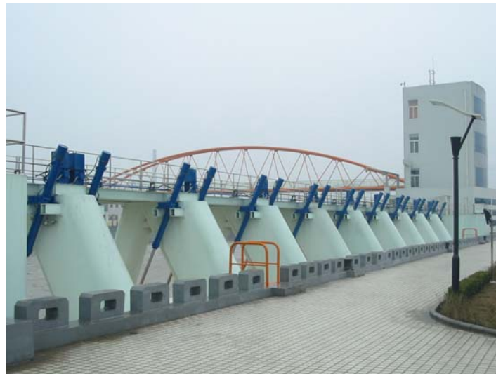
Flood Gate by Bosch Rexroth (20 x RH Profibus)
